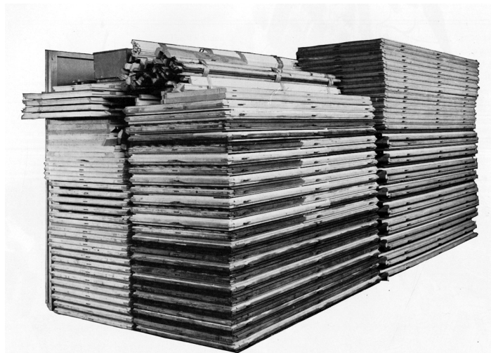
Figs. 144 a, b. Konrad Wachsmann and Walter Gropius, General Panel Corporation, New York, 1943 The packaged house Complete parts of external shell; partitions, floors, ceilings and roof of a four-room family dwelling, prefabricated and delivered in a box, 19' x 8' x 7 1/2' At right is the ground plan showing the basic house with the possible additions when the family is growing.
